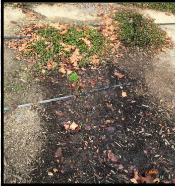
Failed subsurface drip irrigation
