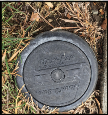
Inefficient pop-up impact spray head
